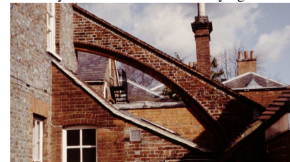
Brick flying buttress on a terraced house
